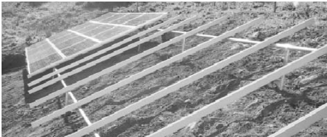
Fig. 12 Ground Trac System by Professional Solar products, showing aluminum support rails, and pipe sub-structure.
