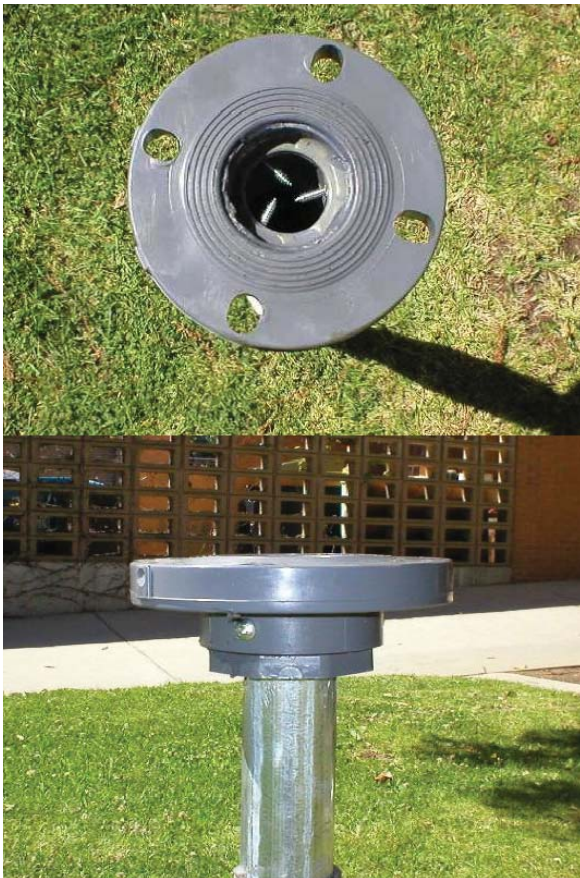
Figure A7. Top and side view of the flange and bushing, showing the #14 × 2" screws that serve as cot pins.
