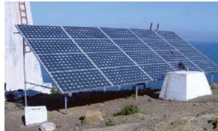
Fig. 14 Solar panels secured to Ground Trac system.
