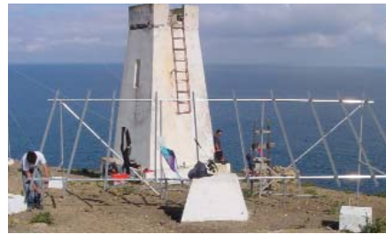
Fig. 13 Ground Trac system being assembled.
